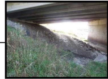
GILES ROAD BRIDGE UNDERPASS - LOOKING SOUTH
