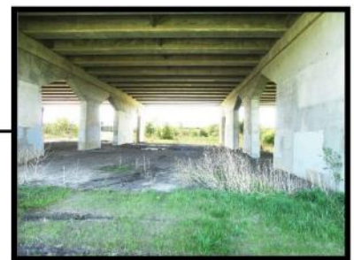
I-80 UNDERPASS - LOOKING SOUTH
