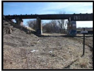
BNSF UNDERPASS - LOOKING SOUTH
