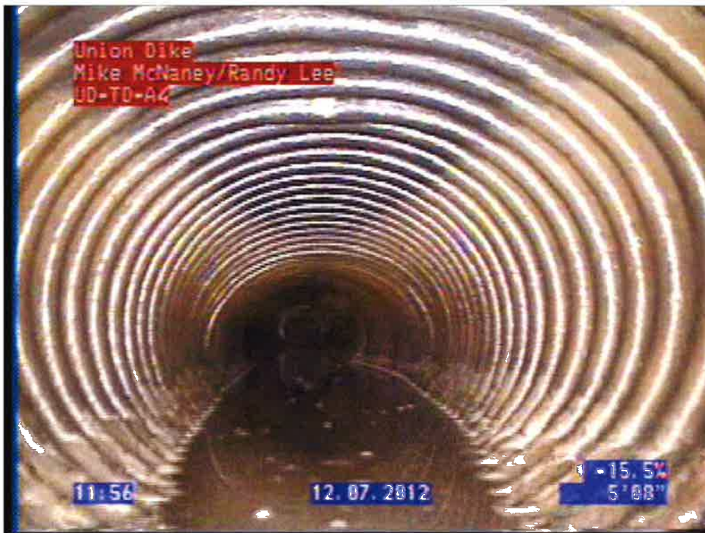
PHOTO 7 - VIEW OF OUTLET A4 - PIPE OUT OF ROUND
