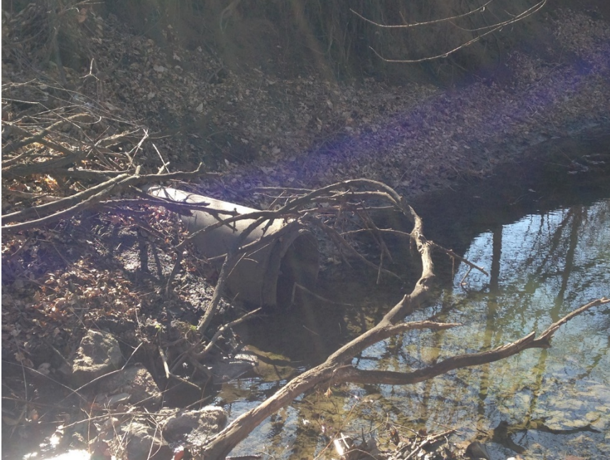
Photo: P6. 18" RCP outlet from apartments.
