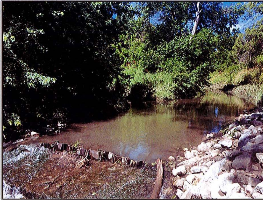
Photograph 4. Looking northwest at flanked grade control structure
