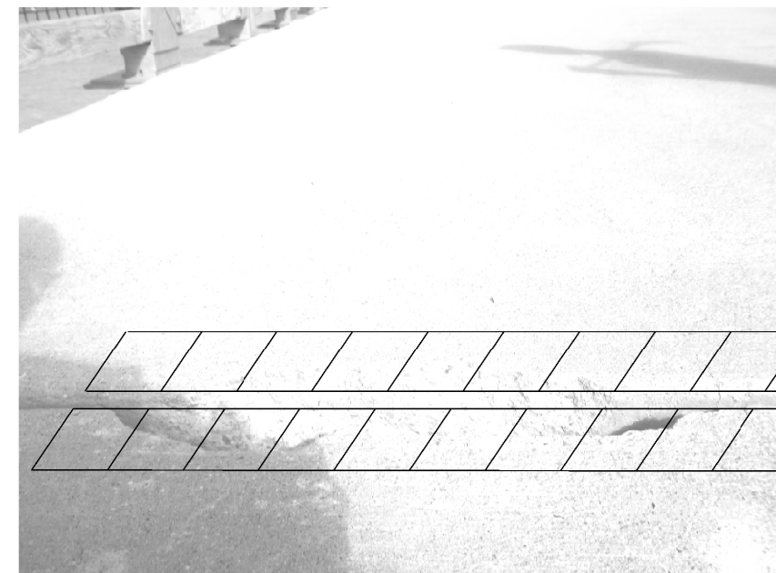
TYPICAL JOINT SPALL
