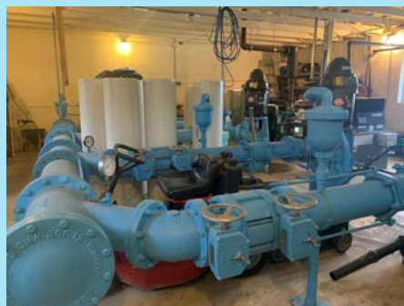
Pipes inside the pump house are connected to three pumps which run on intervals. Each motor runs for 1 week at a time before rotating to the next.
