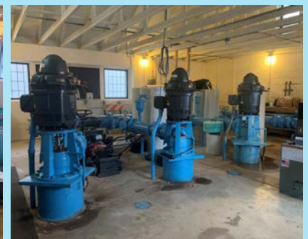
Pipes inside the pump house are connected to three pumps which run on intervals. Each motor runs for 1 week at a time before rotating to the next.
