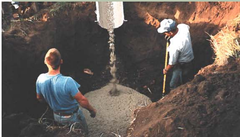
Two licensed water well contractors complete a well abandonment in Washington County.
