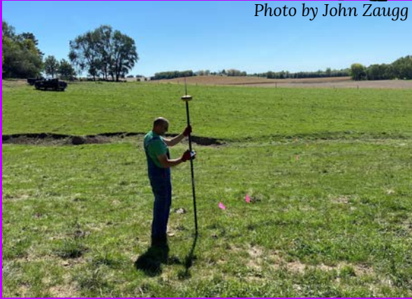
Chuck Venditte, NRCS Soil Conservation Technician, surveys for a Sediment Control Basin near Kennard.
