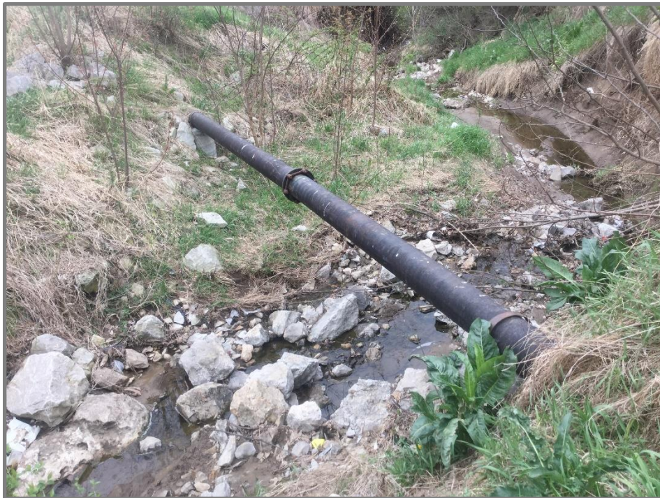
Photo 6. Tributary RS 0140: Aerial 8-inch DIP sanitary sewer crossing located just upstream of confluence with Oakbrook Channel (City Photo taken 4/24/2020).
