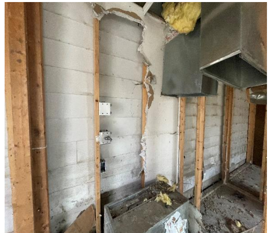
Photo #2 Sample 01: Drywall / Joint Compound Composite Analysis <1% Chrysotile
