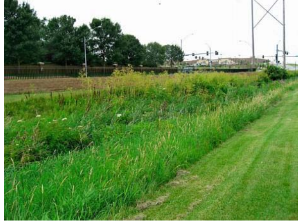
B. Looking downstream toward 72 nd Street (July 2010)
