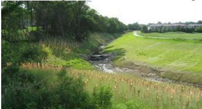
E. Re-graded banks, native vegetation, grade control structures
