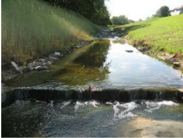
C. Series of cross vane grade control structures
