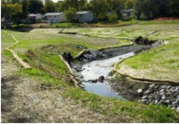
A. Re-graded banks and native vegetation downstream of Sorensen Pkwy B. Cross vane grade control structure and stormwater outfall
