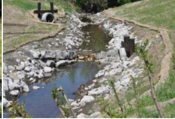
A. Re-graded banks and native vegetation downstream of Sorensen Pkwy B. Cross vane grade control structure and stormwater outfall
