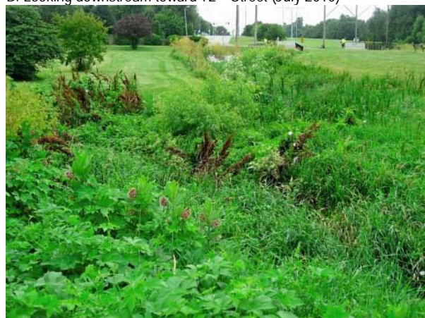
D. Looking upstream from 72 nd Street (July 2010)
