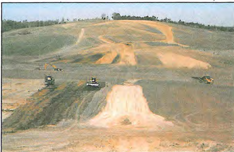
Construction is underway for the stream channel clean out and temporarily diverting Jones Creek while constructing the earthen dam - June 18, 2012.
