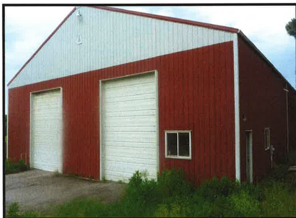
Building 4 – Stable & Equipment Shelter
