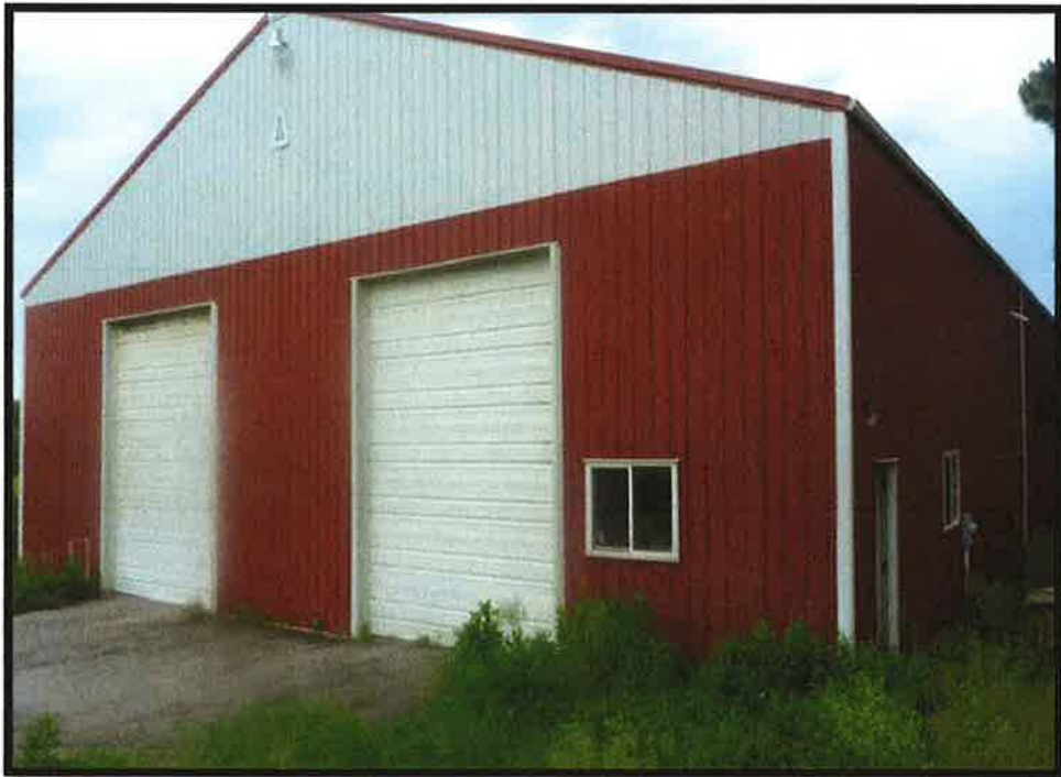
Building 4 – Stable & Equipment Shelter
