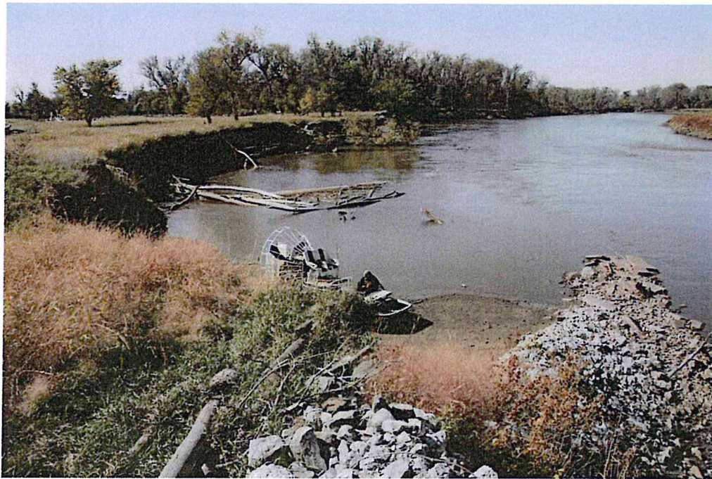
Figure 35. View looking downstream flows from the pre-existing rock spur at Field Site 8 across the scallop in the left bank that developed during the June 2010 high flow.
