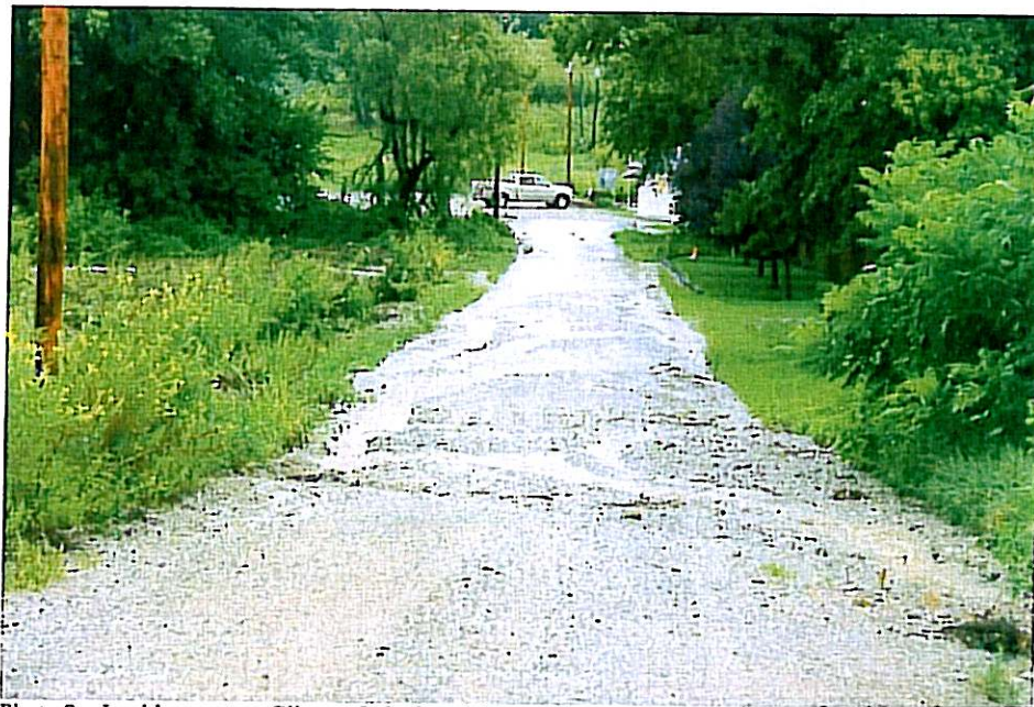
Photo 2 – Looking east on Gilmore Lake Road. Runoff flows from south side to north side of road. (8-19-09)
