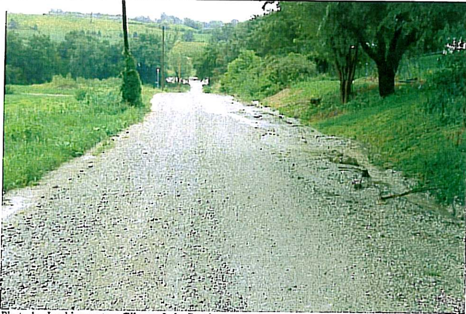
Photo 1 – Looking east on Gilmore Lake Road. (8-19-09)
