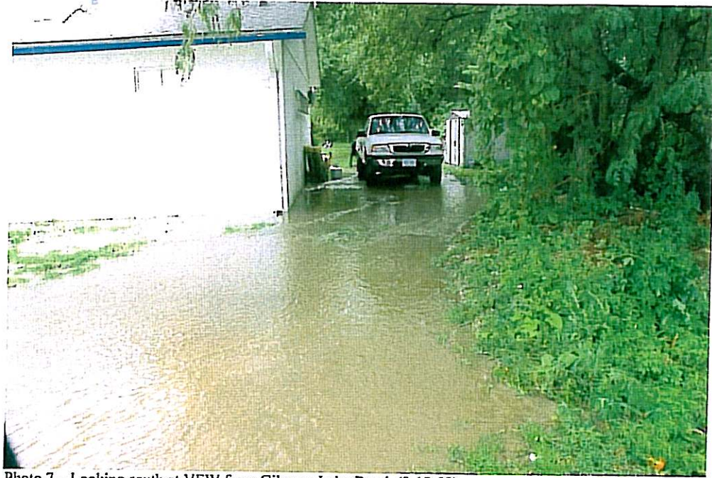
Photo 7 – Looking south at VFW from Gilmore Lake Road. (8-19-09)
