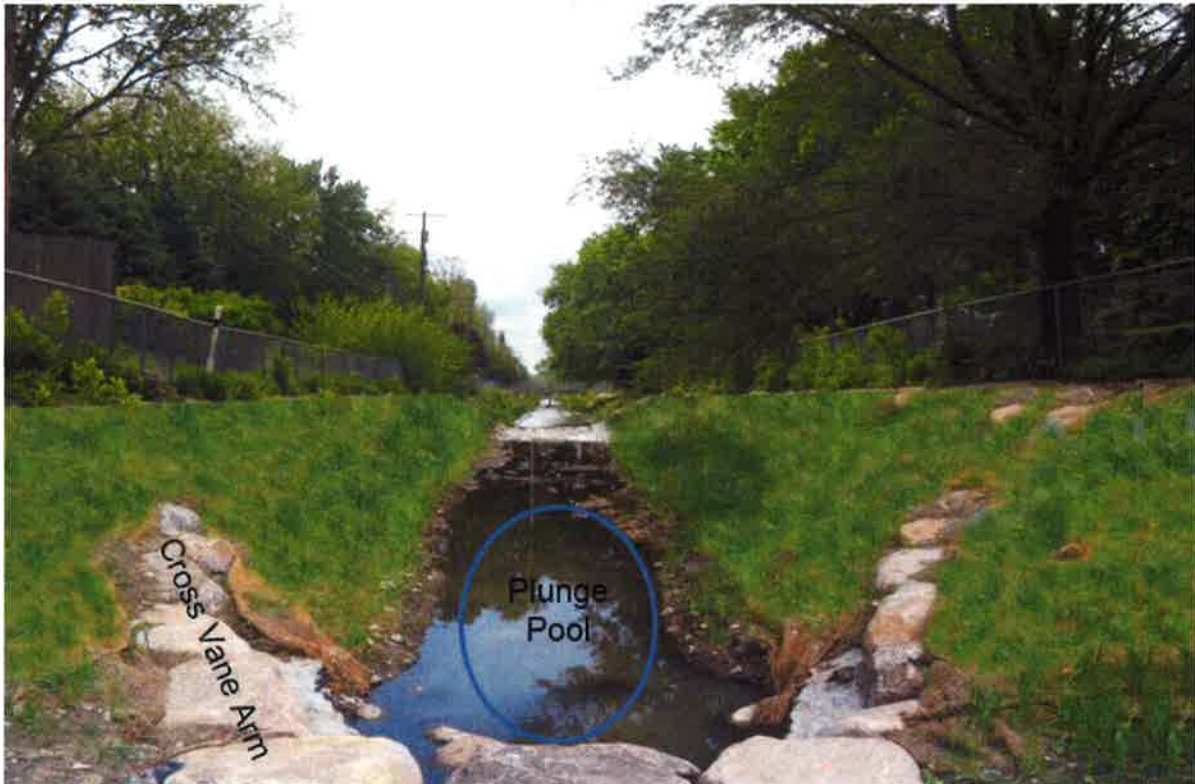
FIGURE 11 –HELL CREEK PROPOSED CROSS VANE ROCK GRADE CONTROL STRUCTURE AND VEGETATED BANKS (CONCEPTUAL RENDERING, LOOKING DOWNSTREAM)
