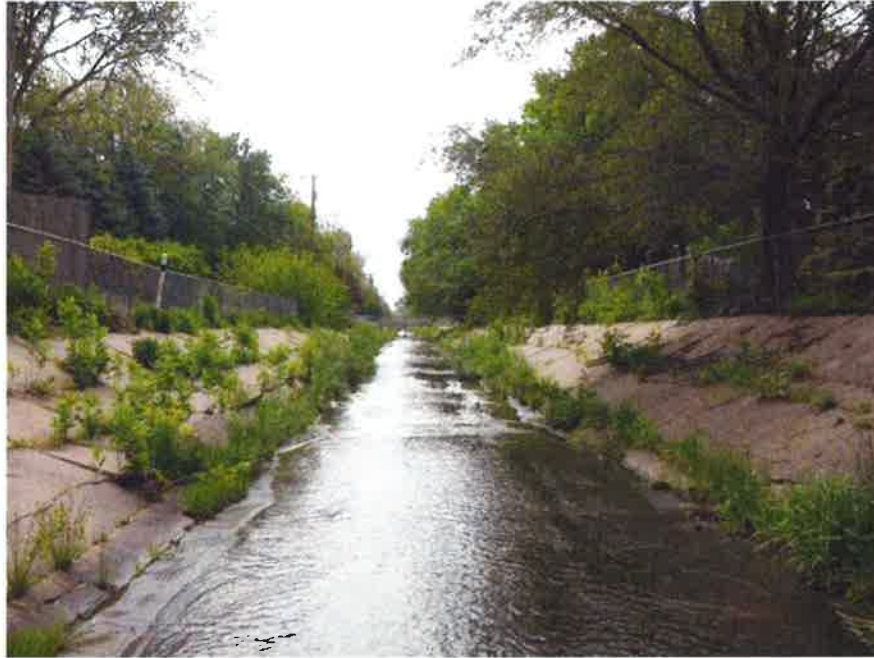
FIGURE 3 – HELL CREEK – EXISTING CONCRETE LINED CHANNEL (LOOKING DOWNSTREAM OF WESTWOOD LANE)
