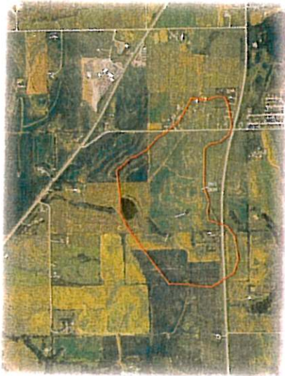
The drainage area protected by the flood control structure is shown outlined in red on the aerial map above. It encompasses over 270 acres.
