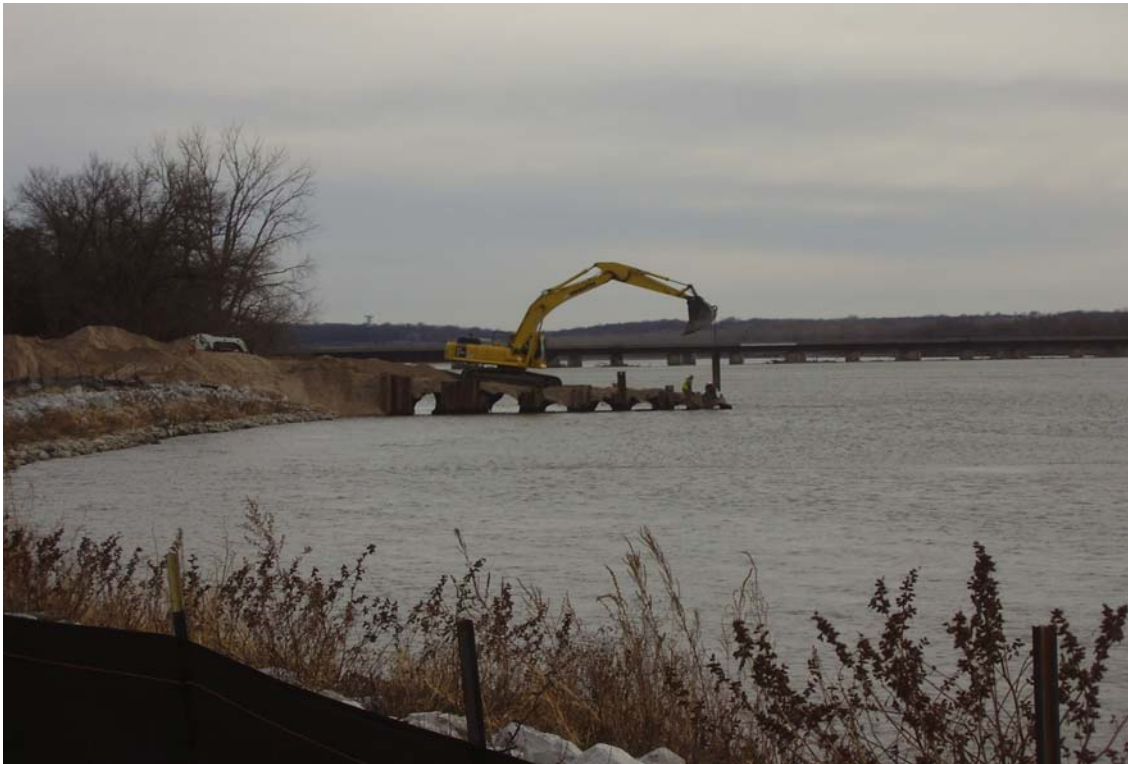
Photo: Construction of the causeway continues. Date: November 28, 2007
