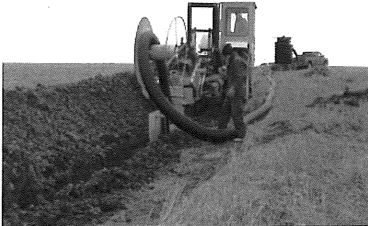
Harry Hauschild is operating the tiling machine as an employee keeps a close eye on the progress. The risers are offset 4 feet off the tile line in each terrace channel.
