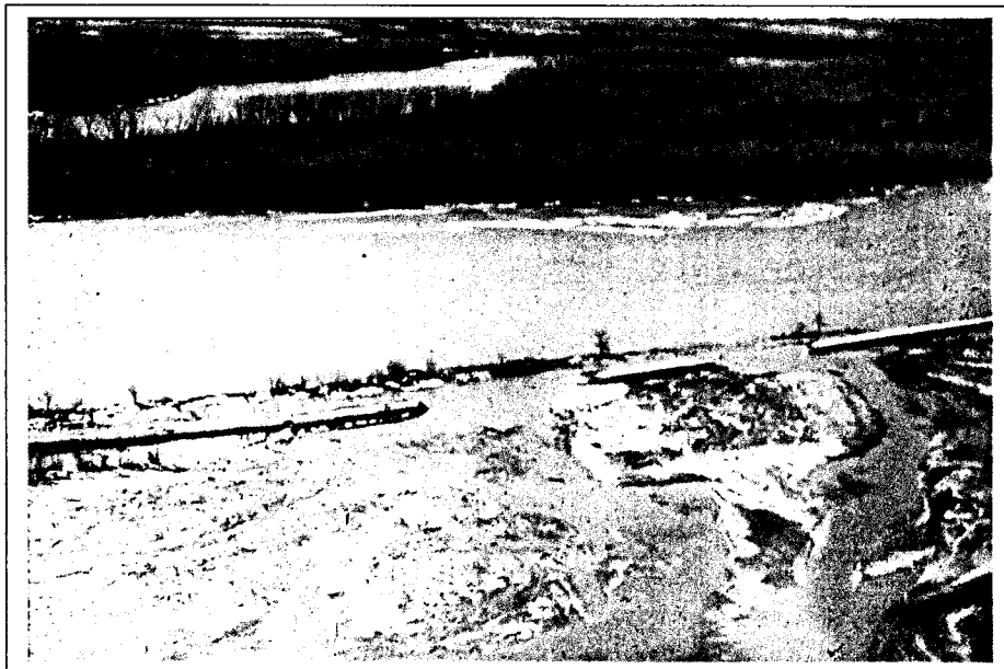
Photo 4. View of breaks in Union Dike during the 1978 ice-jam flood event.
