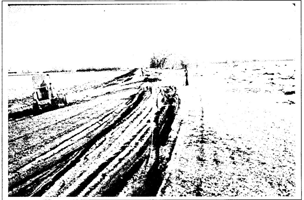
Photo 5. View of the ice jam on Platte River adjacent to Union Dike. Note water overtopping the levee.
