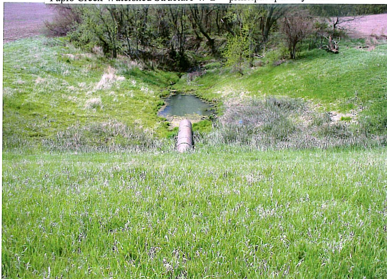
Papio Creek Watershed Structure W-2 ---principal spillway outlet
