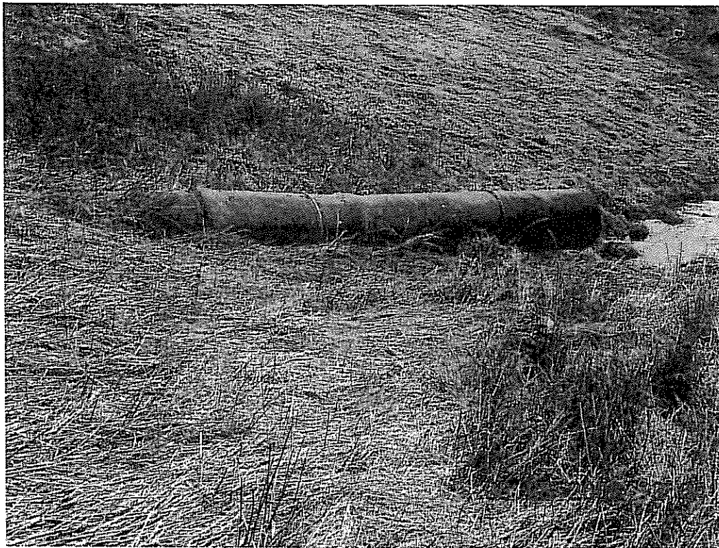
View of Pipe Distress in Principal Spillway
