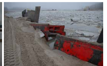
Use of trench boxes to reinforce causeway
