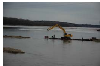
Building north causeway
