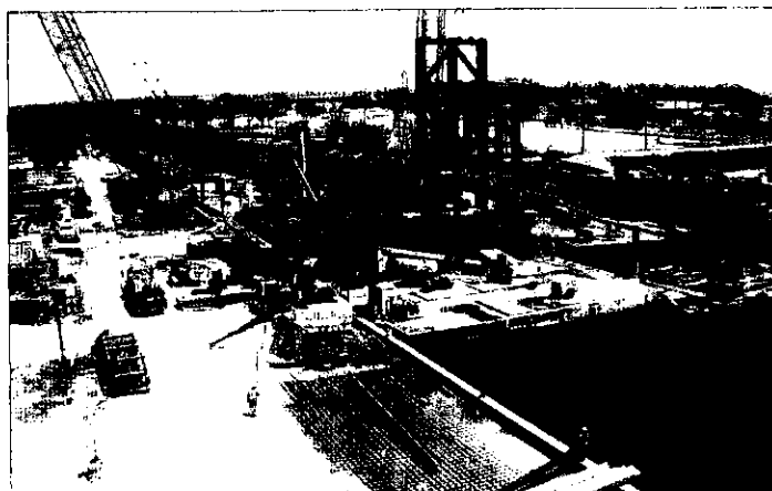
▲ Relentless. Contractor crews set jacket for temporary canal gate.
