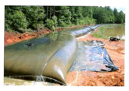
Geotextile Dewatering Tubes, Also referred to as Sludge Tubes, Geo-Tubes (short for geotextile), Dewatering Tubes, are ideal for filtering materials on projects and are used extensively on Water Treatment projects (WWTP's), agricultural ponds, aquaculture facilities, pulp and paper mills and numerous industrial lagoons for consolidation of media.
